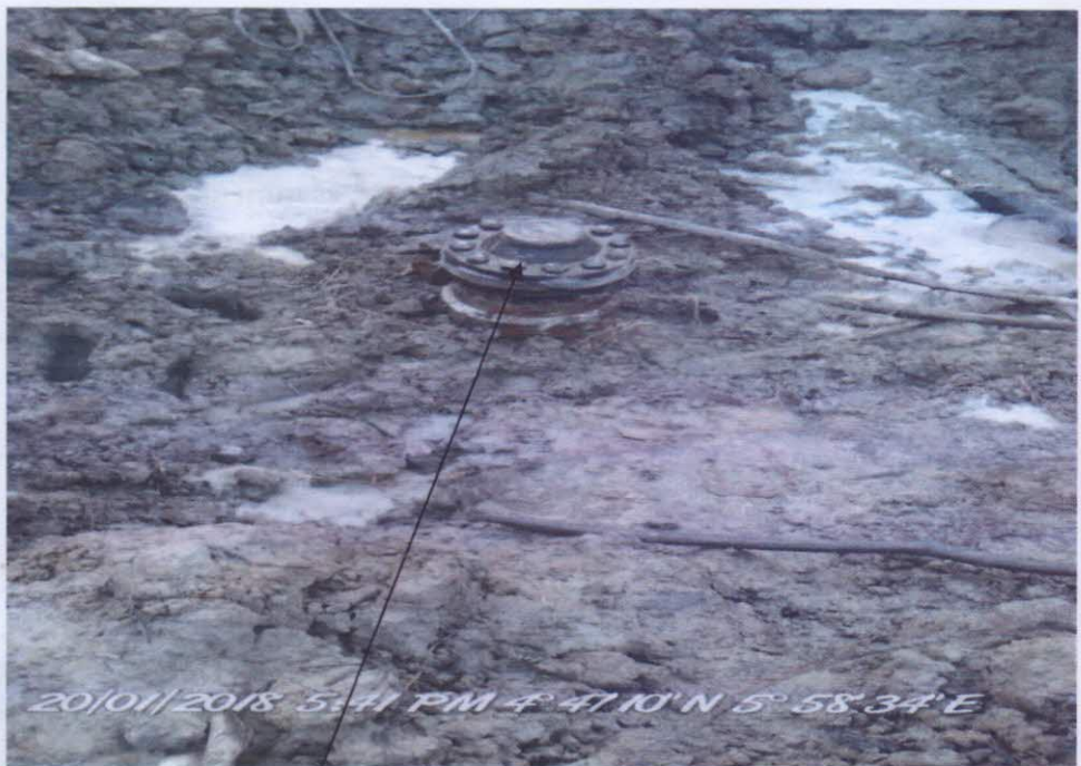
Spill Leak Point After Repairs.
